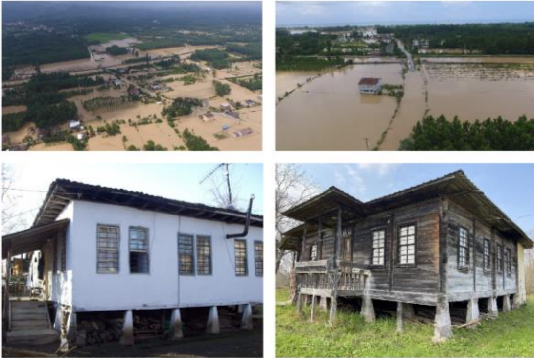
Photo 7. Flood disaster in the Çarşamba Plain - Yeşilirmak Delta on June 22, 2019 (Source: DHA). Two examples of delta houses built on poles high above the ground, very few of which have survived to the present day in case of similar problems in the past.
