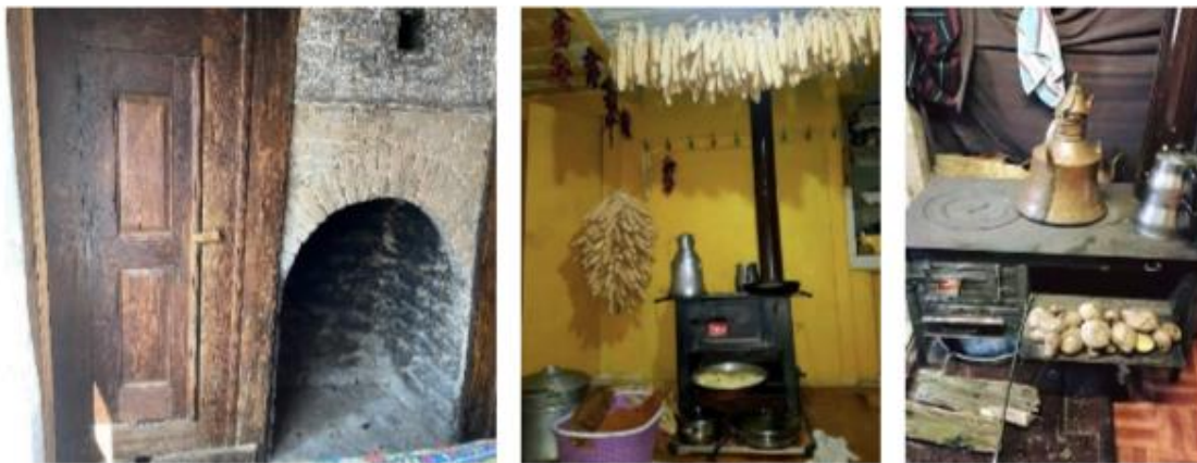
Photo 4. Fireplace and rovine stoves are used to heat homes while cooking and drying at the same time, saving energy.
