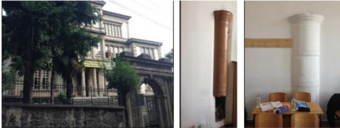
Photo 5. A stove system in an old school in Giresun, where a single stove heats two adjacent classrooms.
